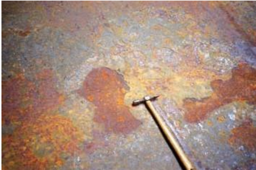
Loose scale must be removed from the tank top before grain loading
