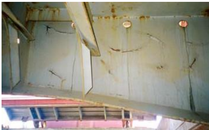
Flaking paintwork under the hatch coaming can result in a hold failing the grain survey
